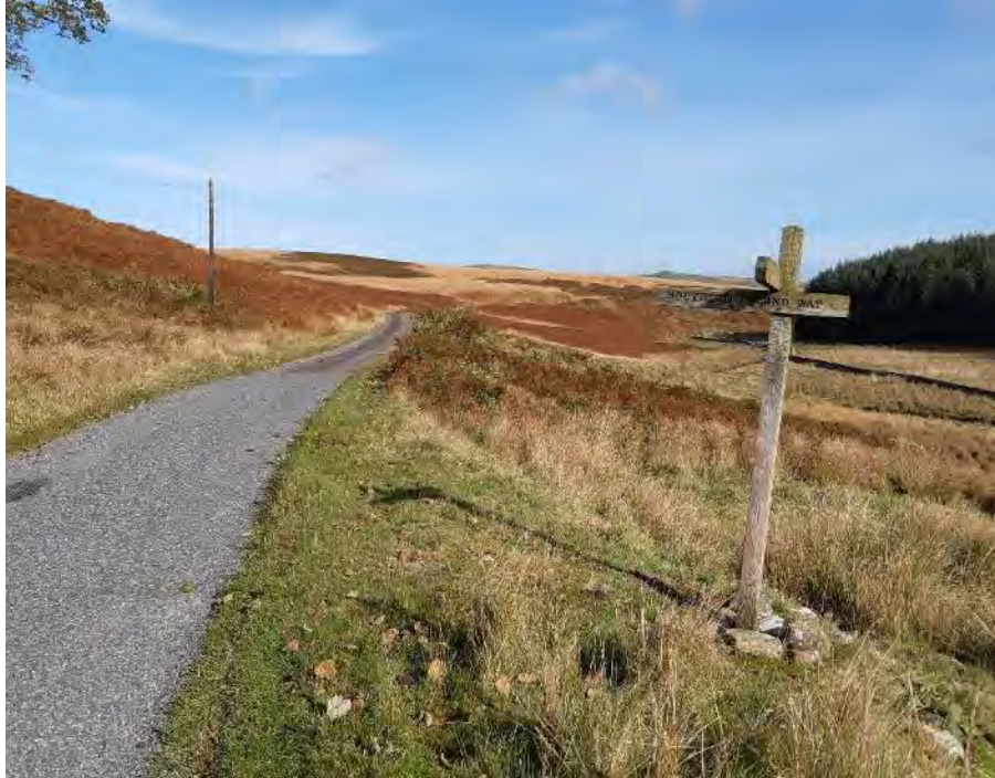
Figure A4.7.3: SUW at the intersection with the National Byway Cycle Route and the Fingland Lane
